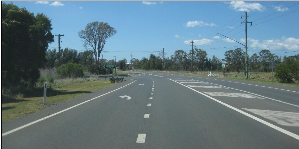
Figure 2.9: Luddenham Road/Elizabeth Drive Intersection – viewed from Elizabeth Drive west
